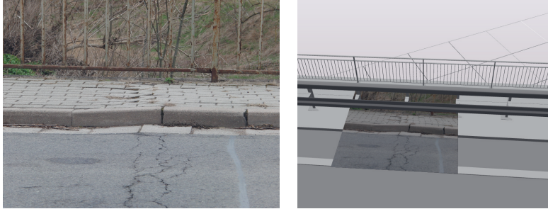
Figure 5.11: Representation of some cracks at the pavement as a texture depicted on a plane.
