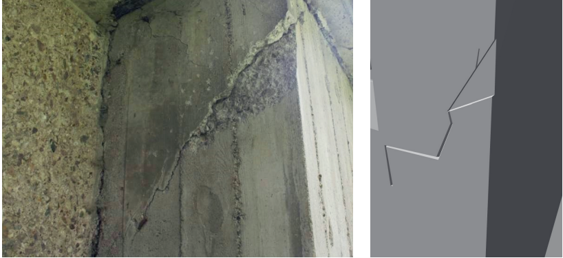
Figure 5.12: Representation of a spalling at the abutment.
