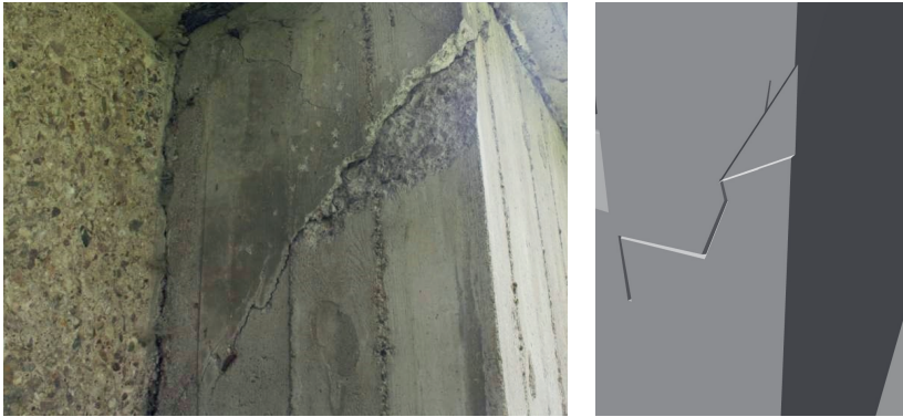
Figure 5.12: Representation of a spalling at the abutment.
