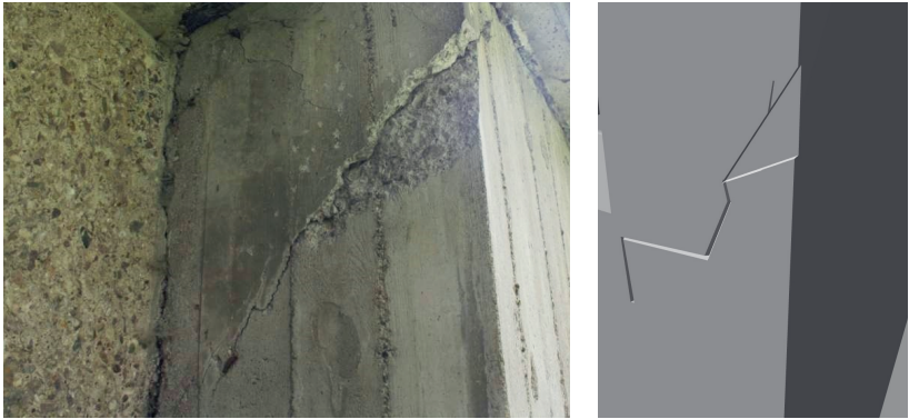
Figure 5.12: Representation of a spalling at the abutment.
