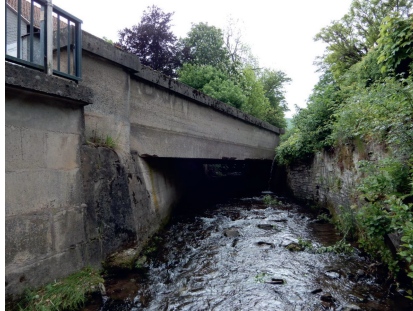
Figure 5.6: Photo of the bridge for case study. The photo has been provided by the "Thüringer Landesamt für Bau und Verkehr".
